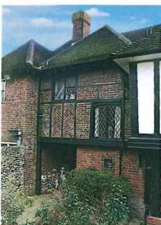
Figure 3. The porch bay on the north-west side of Poynings: the front door is hidden within the recess. Ranger occasionally designed half-timbered sections of wall that looked as if they reused old materials (Timothy Brittain-Catlin)
