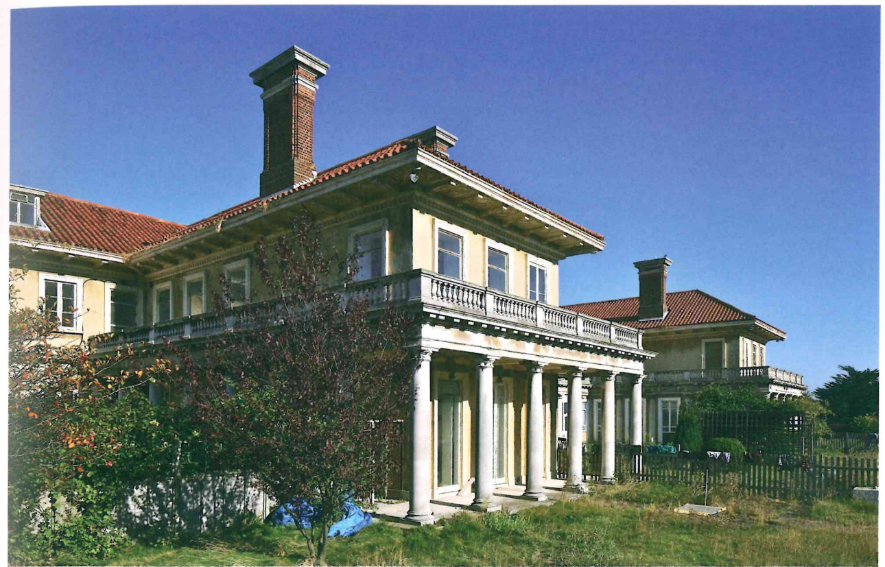
Figure 10. Thanet Place, a large house on a relatively small site designed in collaboration with Sir Charles Allom. This view from the west shows part of the garden front just before the recent conversion of the building into flats (John East)
