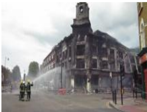
Figure 2.1: Originally built by the London Co-operative Society in 1930, in 2011 this building included a Carpetright store and flats on the upper levels 82
