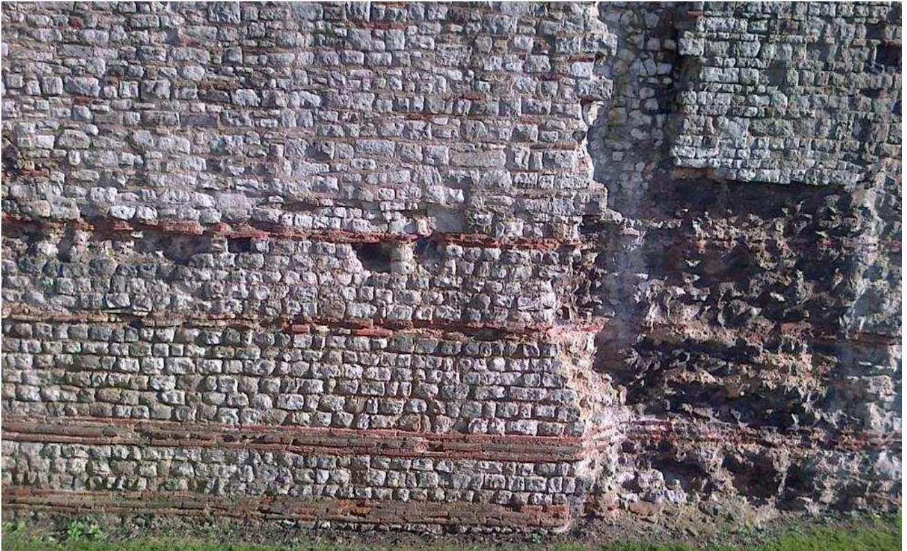
Figure 1: Finely worked upper Medway Valley Kentish ragstone blocks in the land wall of Roman London (this location near Tower Hill), late 1 st century AD. Hall and Merrifield (1986, 28) said over one million squared and dressed ragstone blocks, from the five quarries identified for the first time in this research, would have been used for the inner and outer facing alone. Simon Elliott.
