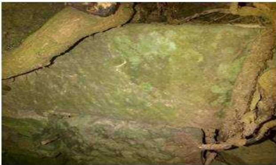
Figure 69: Re-used ragstone lintel from Teston villa site, river wall at Teston Medieval oil mill. Simon Elliott.
