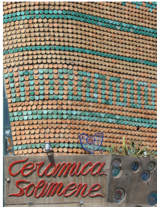
5.2.3. Detail of the façade (current condition)
