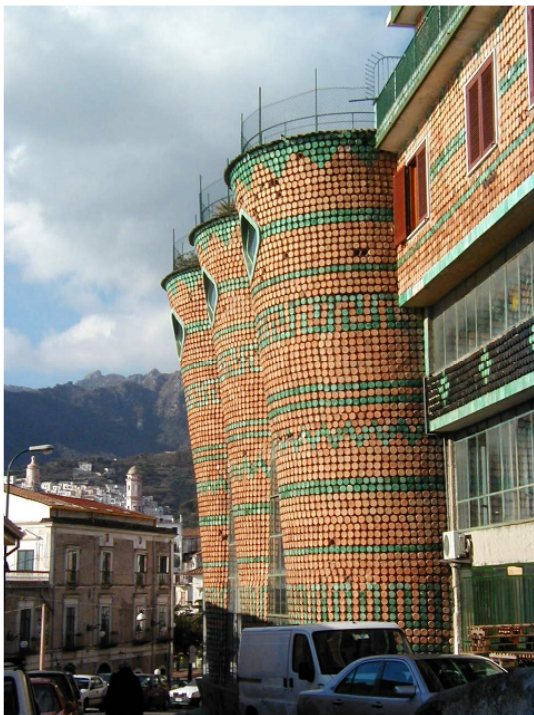
5.2.2. External view (current condition)
