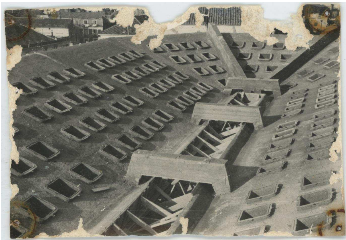
Figure 5. Solimene Ceramic Factory, Vietri sul Mare, 1956, Architect Paolo Soleri. The funnel-shaped skylight with the \Pi -shaped connections at the top of the frame. (Photo: Cosanti Foundation – Colly Soleri, Soleri Archives collection.)
