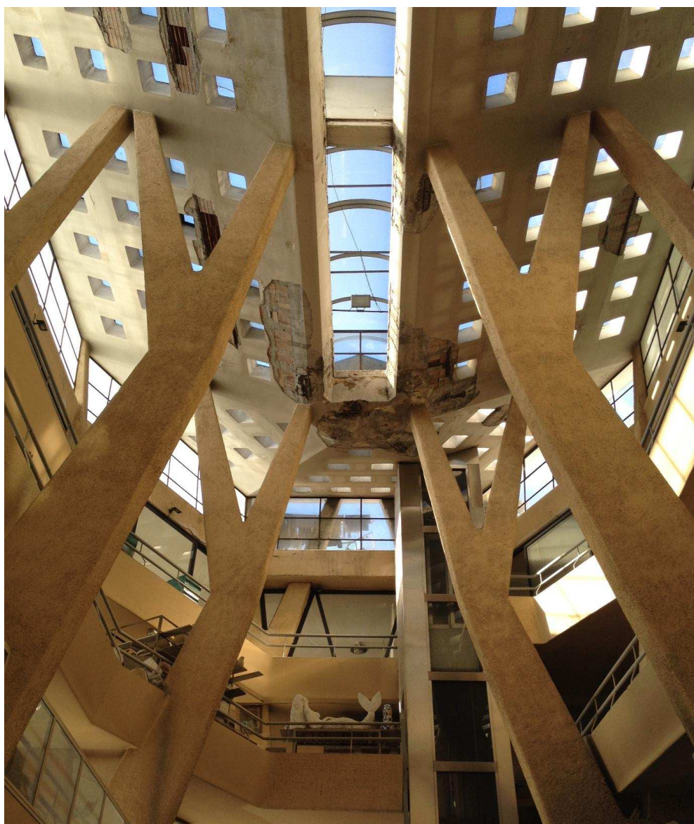
Figure 14. Solimene Ceramic Factory, Vietri sul Mare, Salerno, 1956, Architect Paolo Soleri. The present state of the production hall with the new elevator put in place and the plaster cracked on the roof (January 2016). (Photo: Luciano Cardelicchio)
