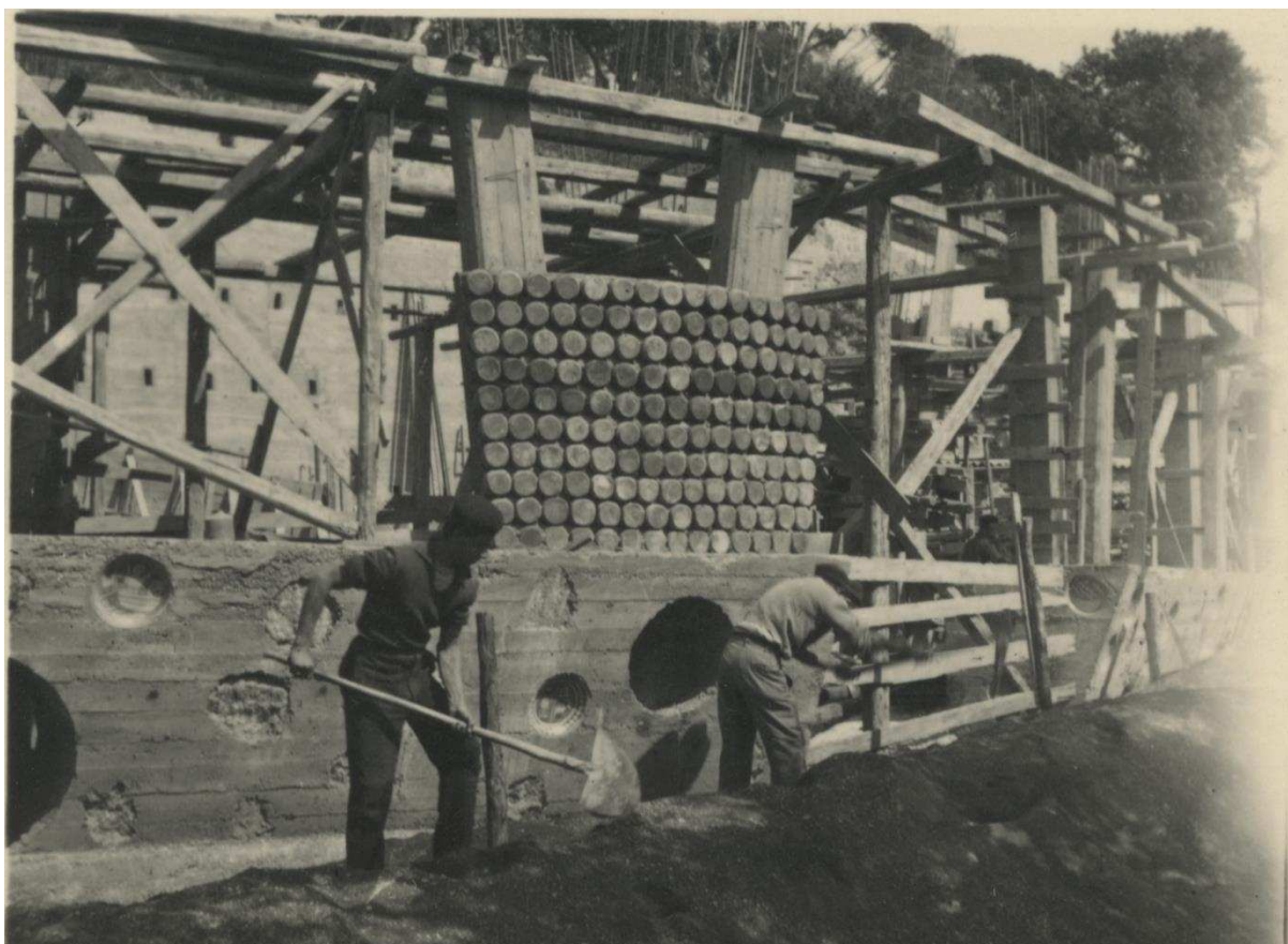
Figure 8. Solimene Ceramic Factory, Vietri sul Mare, 1956, Architect Paolo Soleri. The first mock-up of the fictile external wall in 1953. (Photo: Cosanti Foundation – Colly Soleri, Soleri Archives collection.)
