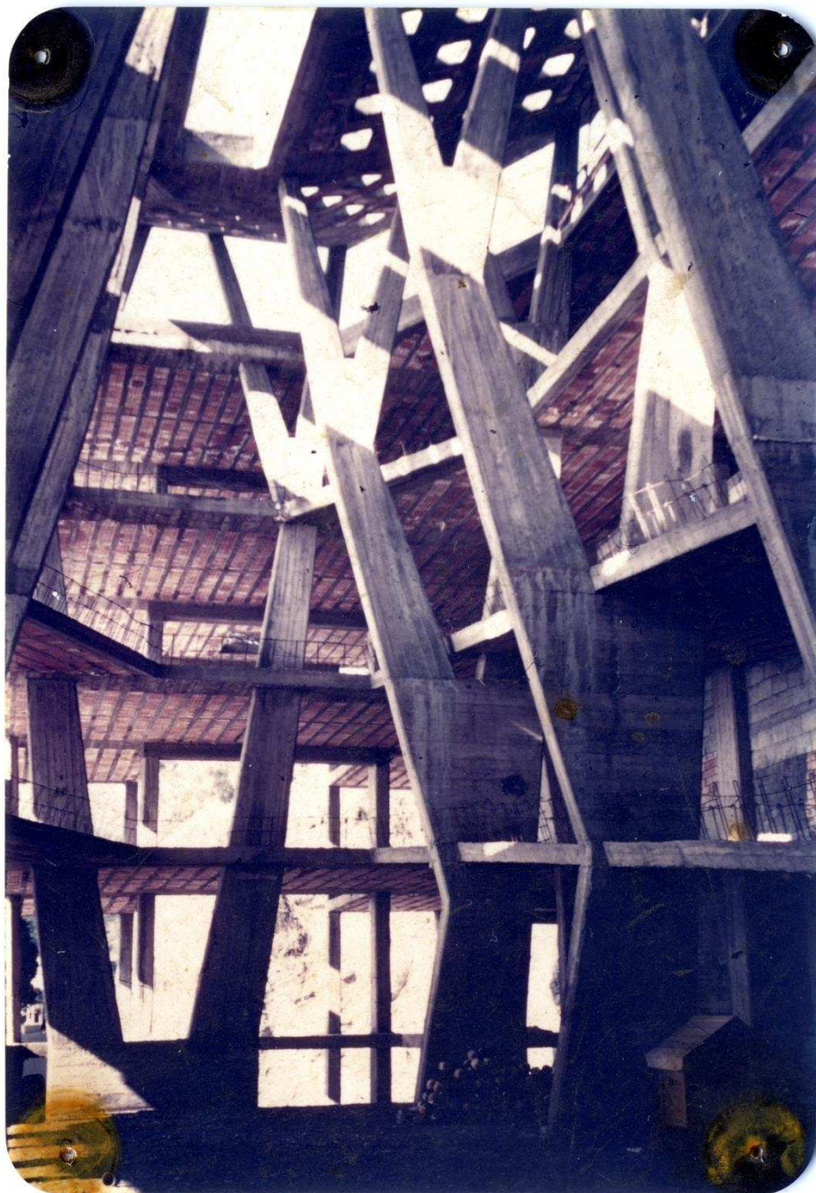
Figure 4. Solimene Ceramic Factory, Vietri sul Mare, 1956, Architect Paolo Soleri. The production hall with the two types of tree-shaped columns. (Photo: Cosanti Foundation – Colly Soleri, Soleri Archives collection.)
