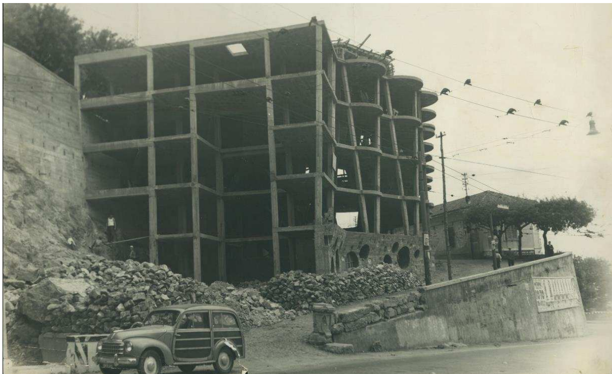
Figure 6. Solimene Ceramic Factory, Vietri sul Mare, 1956, Architect Paolo Soleri. The structural frame of the production hall by the quadruple-high space for the vertical wooden pot-kiln. (Photo: Cosanti Foundation – Colly Soleri, Soleri Archives collection.)
