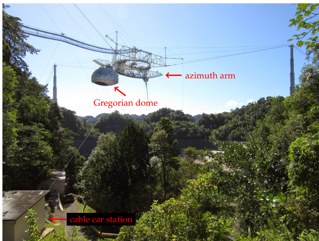
Figure 5.3: The Gregorian dome of Arecibo telescope hangs about 137 m above the 305 m primary mirror. It is attached to a rotating azimuth arm suspended from a triangular platform. The dome hosts secondary and tertiary mirrors, as well as a wide range of instruments, including the S-band radar transmitter and receiver, which can be accessed after a short trip with the cable car or a walk up a narrow bridge. As the telescope's primary mirror is not movable, the Gregorian dome can be slid along the azimuth arm to control the elevation at which objects are observed and the whole arm can be turned to adjust azimuth. The photograph was taken from the perspective of the control room by A. Rožek during her observations in January 2015.
