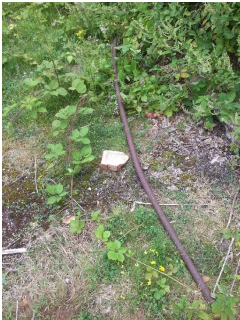
Fig. 4 Example of metal tubing used as a buried spraying system
