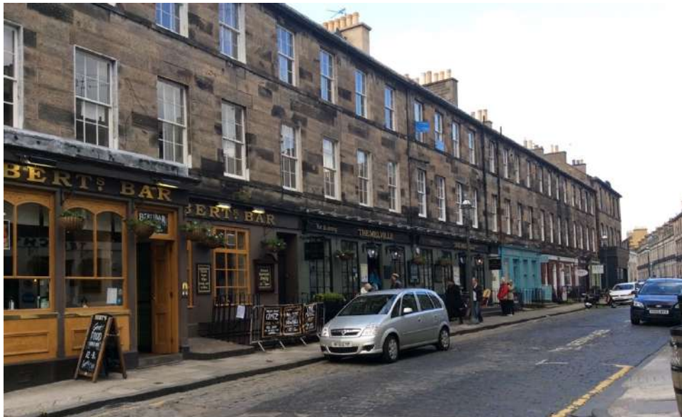
Figure 38: Example of ashlar-faced architecture in the New Town of Edinburgh. © Francesca Giliberto
