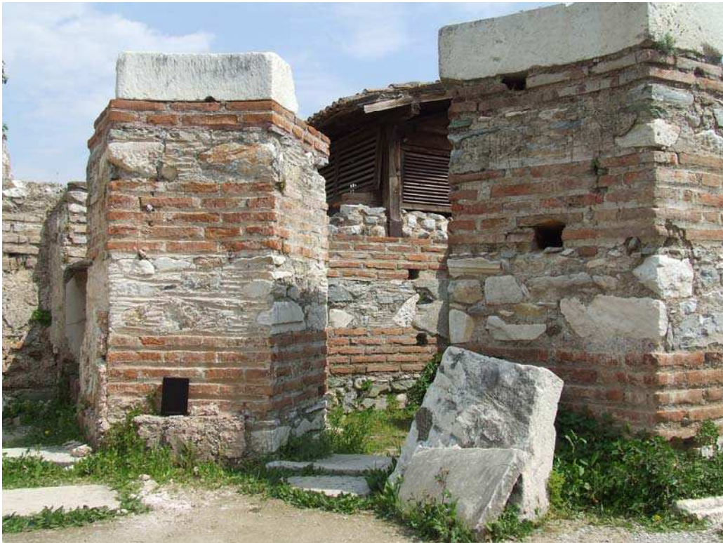
Figure 11. View of the central piers of the skeuophylakion
