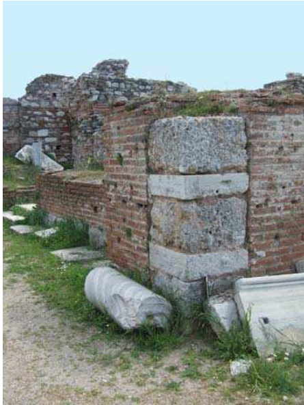
Figure 19. Detail of the junction between the northeast external walls of the transept and the north external wall of the east cross arm.
