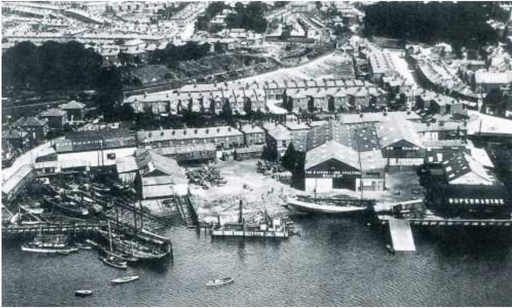
Figure 12. Aerial view of the Supermarine Factory, Woolston, (1919)
