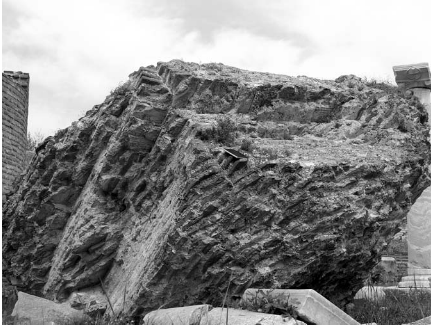
Figure 12 St. John at Ephesos, vault fragment C, view from the southeast, showing remains of supporting arches (with double arch-rings) and vault core (author's photo)
