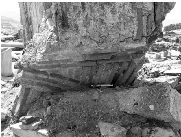
Figure 7 St. John at Ephesos, detail of vault fragment A, showing remains of supporting arch and pendentive. The pendentive is flanked by two borders consisting of three brick courses (author's photo)
