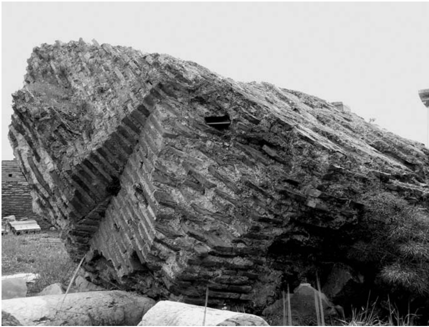
Figure 14 St. John at Ephesus, vault fragment C, view from the northwest. Note the intersection between pier and broad arch on the left part of the figure (author's photo)
