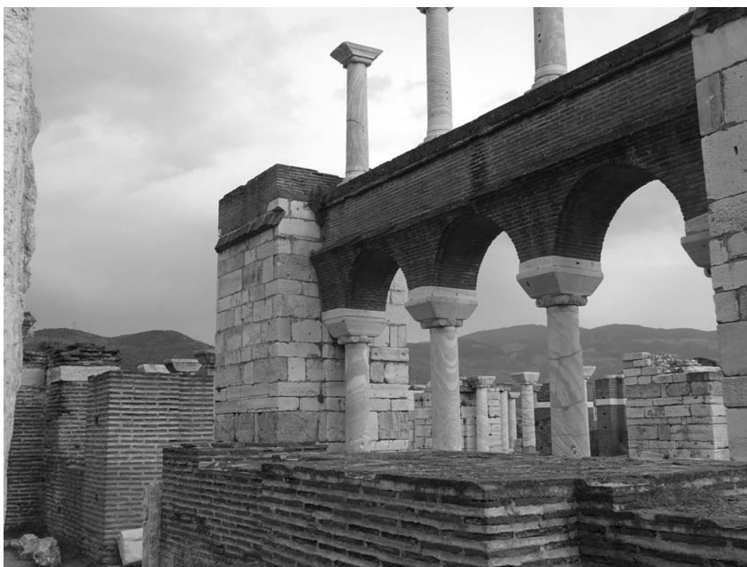
Figure 23 St. John at Ephesos, nave, mid-twentieth-century partial restoration of the south colonnade (author's photo)
