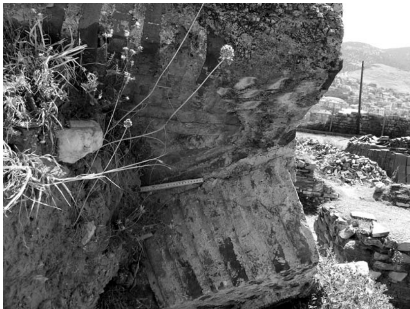
Figure 9 St. John at Ephesos, vault fragment B, view from the west. Detail of the convergence of two broad arches, showing the springing of a pendentive between them (author's photo)
