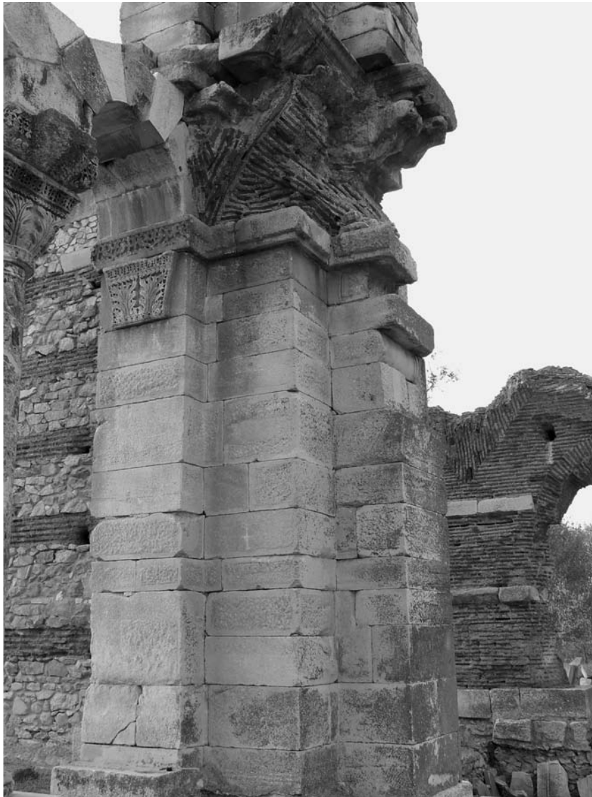
Figure 21 Basilica B at Philippi, detail of aisle vault fragment, showing remains of the gallery floor (author's photo)
