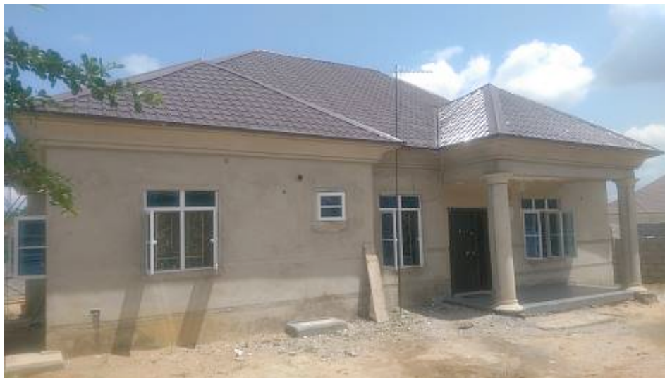
Figure 3: Front view of Case Study 1
