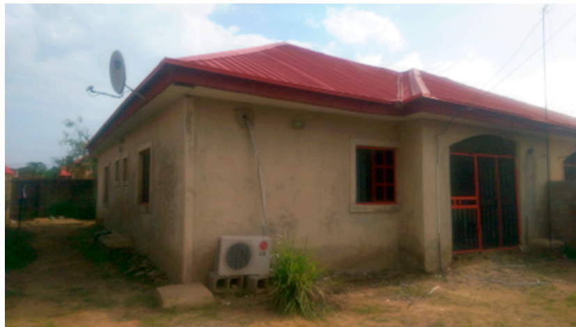
Figure 5: Main building, Case study 2
