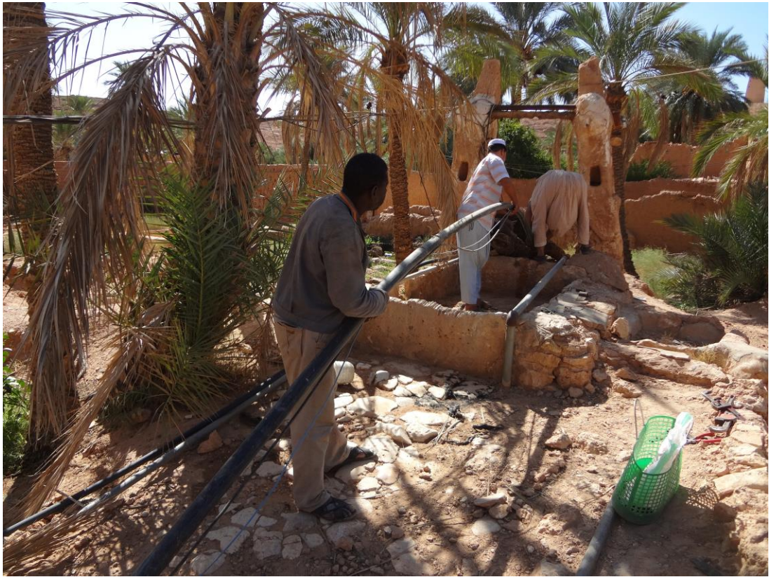
Figure 4.8 Plumbers repairing an immersion pump in an artisanal well. (29/10/13)
