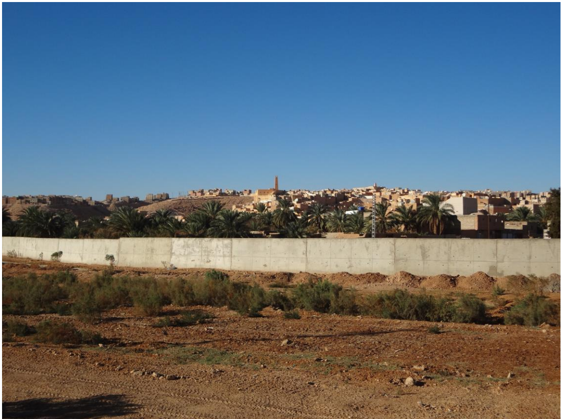
Figure 8.2 New state-built concrete walls on the edge of the river. (03/11/13)
