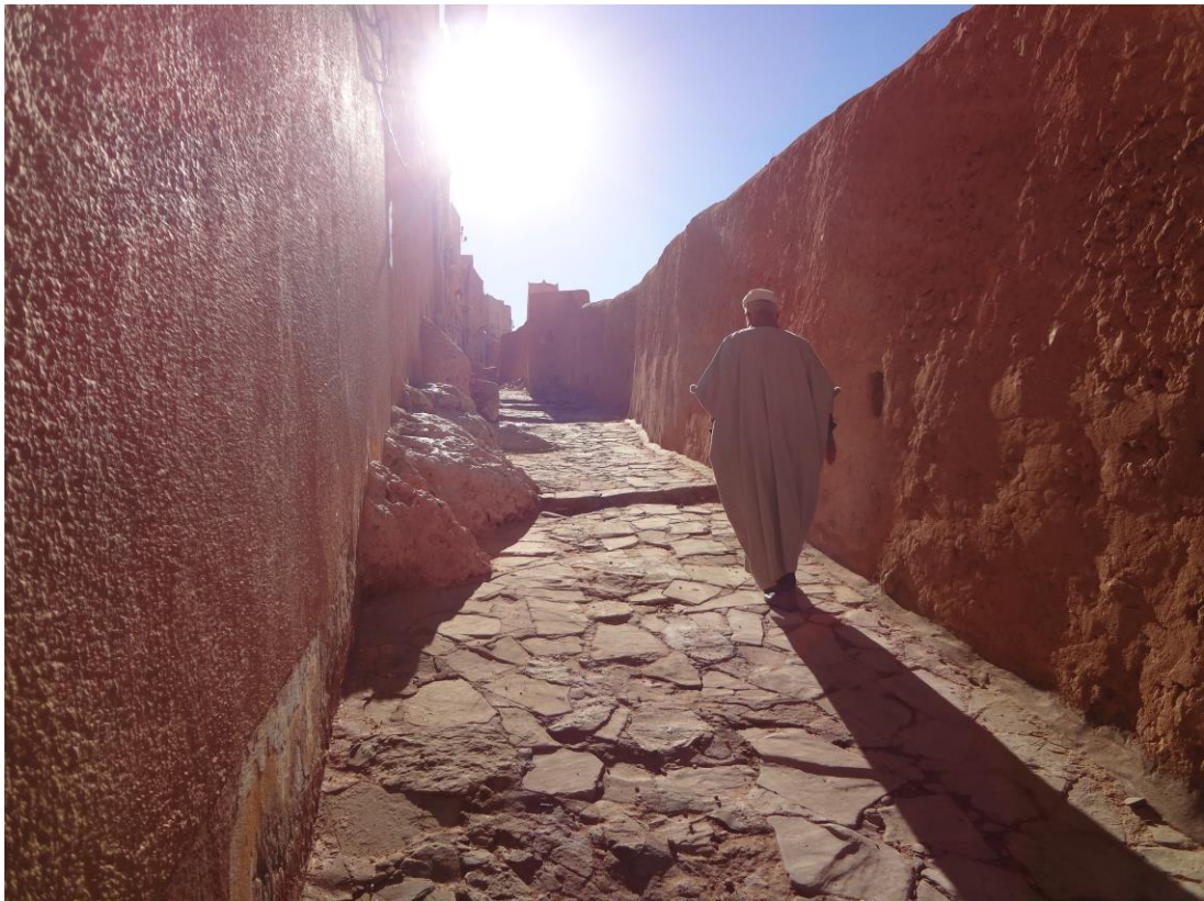
Figure 4.4 Inside the outer wall of the Beni Isguen. (19/12/12)
