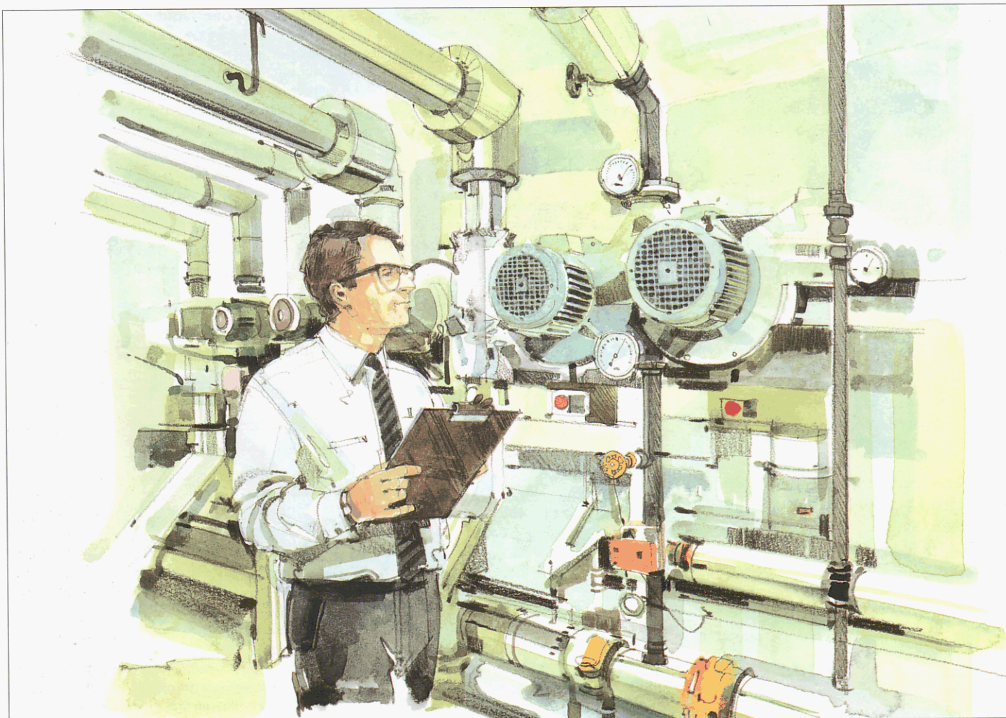
Ensure that all pipework including insulation, valves and flanges are checked regularly
