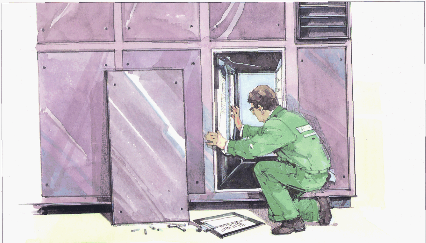
Rotary heat exchangers require routine inspection
