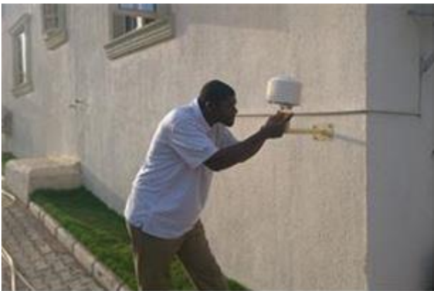
Fig 5: Installation of Tiny Tag external data loggers
