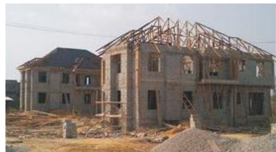
Fig 2: Building construction in Nigeria
