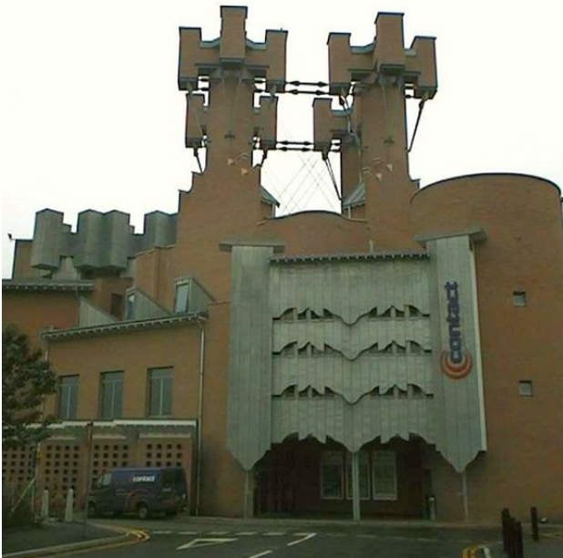
Fig 2: The naturally ventilated Contact Theatre, UK
