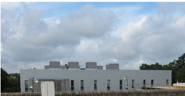
Fig 3: The ventilation stacks of the Jarman building
