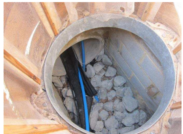
Fig 4: Junction of manhole and earth tube
