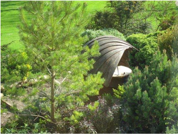
Fig 2: Cowl above inlet to earth tube
