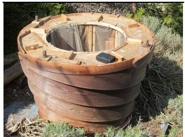
Fig 3: The air inlet terminal above the manhole
