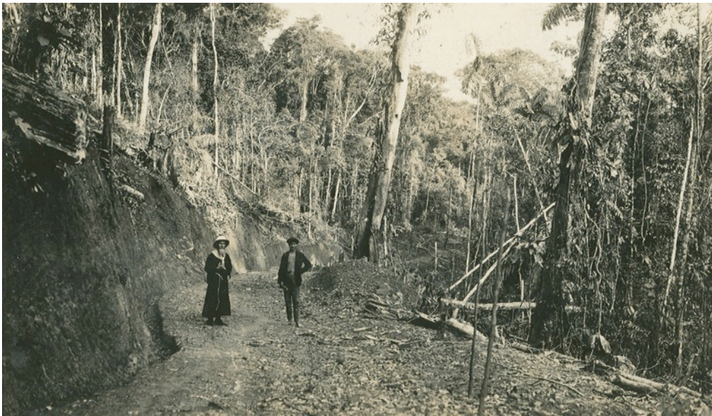
Figure 2. 1909-1930 Puerto Umbría –Puerto Asís Road construction led by the Capuchins (CEPAC)
