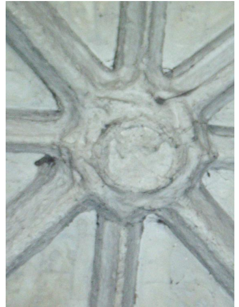
Fig. 1.11: Present day condition of the boss where the coronet is just discernible.
