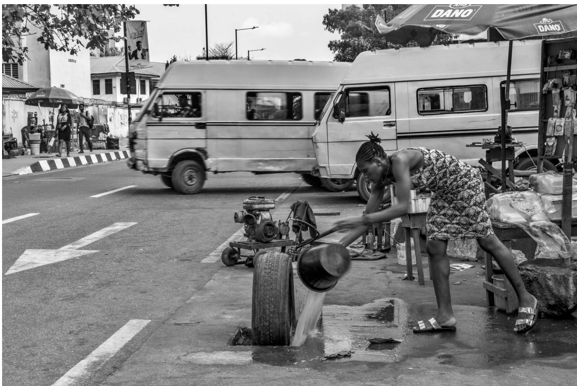
FIGURE 9. Old tyre used to cover a missing manhole.
