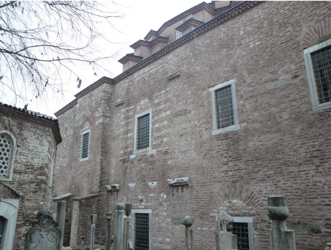
Sergius and Bacchus: Extensive Evidence of Previous Alterations on the External Walls, which include significant portions of Ottoman and Middle Byzantine Masonry
