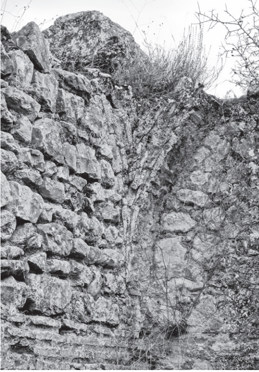
Fig. 2. NE Baths of the Sanctuary of Asklepios at Epidaurus: pendentive remains in Room F1 (need source ).
