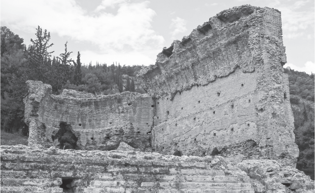
Fig. 1. The Great Hall of Bath A at Argos: view from the south (need source ).
