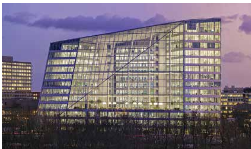
▼ Finalized in 2015, the Edge building in Amsterdam, also known as “The Computer with a Roof”, is equipped with 28,000 sensors that utilize data generated by building users to optimize space management and occupation levels.
