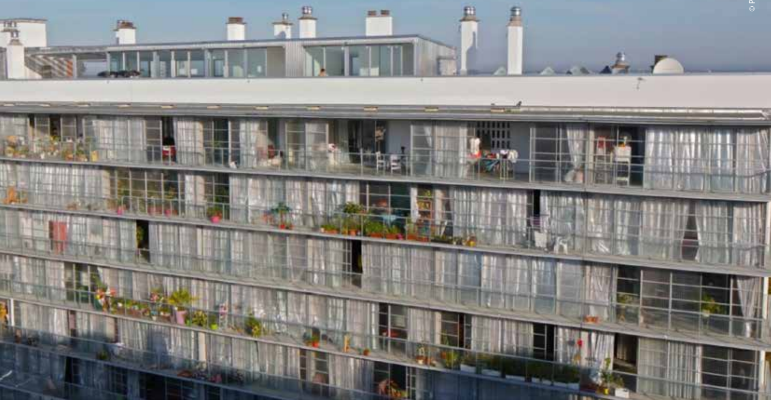
▼ The Grand Parc project illustrates how an overlooked structure can be transformed into comfortable and energy-efficient housing. This transformation cost three times less than demolishing the old building and constructing a new one.
