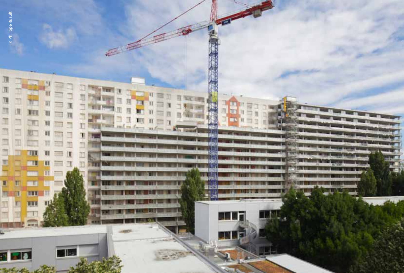
▼ The transformation of three buildings in the Grand Parc housing complex in Bordeaux (France) by Lacaton & Vassal, Druot, Hutin in 2017. The apartment blocks dating back to the 1960s were upgraded with winter gardens.
