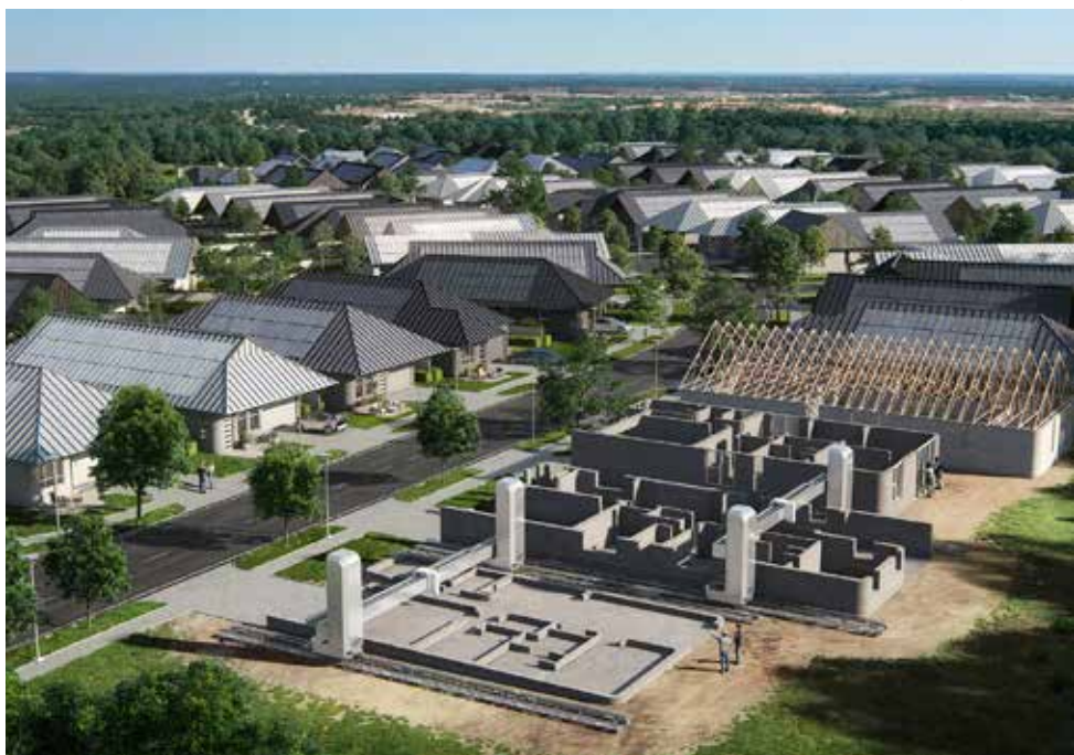
▼ The largest automated 3D construction project in the world is currently underway in Georgetown, Texas (United States): a neighbourhood of a hundred houses.
