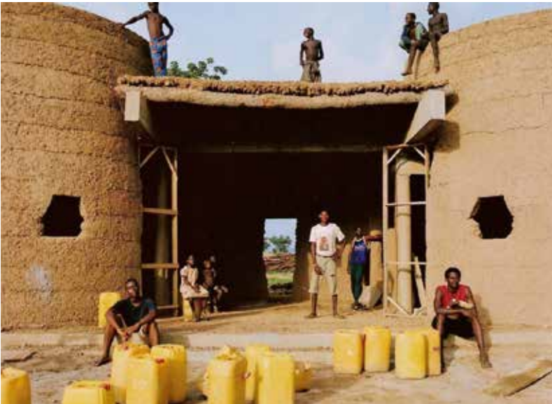
▼ Sénamé Koffi Agbodjinou (front right) on the Tammari school construction site in 2006. The school was built using local raw earth construction techniques.
