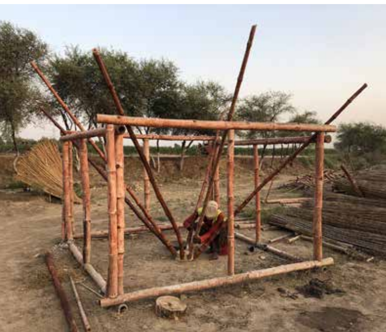
▼ A young artisan learning to build the conical-shaped roof of a chaunra (one-room house) in Bhoriyoon village in Pakistan.
