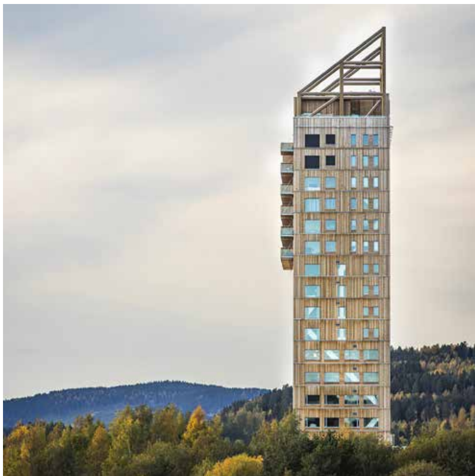
▼ Inaugurated in Brumunddal (Norway) in 2019, Mjøstårnet ("the tower of Lake Mjøsa") is one of the world's tallest timber buildings, standing over 85 metres high.
