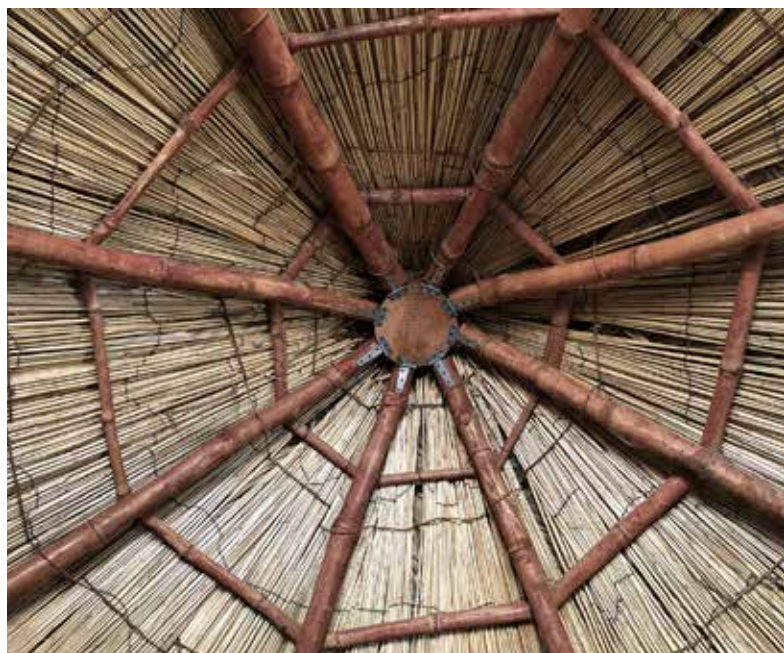
▼ The inside of the octagonal roof of the chaunra , made of bamboo and thatch.
