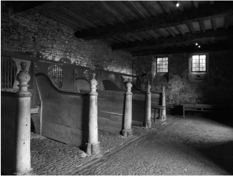
Fig. 10: Nineteenth-century tie stalls in the seventeenth-century stables at Dunster Castle, Somerset. Photograph: C. Hopkins
