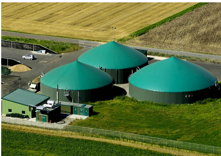
Figure 2 - Anaerobic Digestion Plant, located in Ireland (11).
