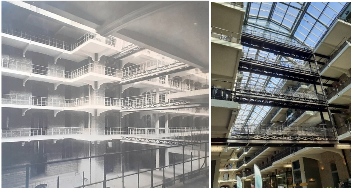
Figures 3.15 (a) and (b): Entrepôt Royal B import warehouse, Brussels (van Humbeek, 1906) after construction in 1906 (left) and the renovated building today (right), showing the daylit atrium with cantilevered galleries made from béton armé . (076 Ifa 54/15. CNAM/SIAF/Cité de l'architecture et du patrimoine/Archives d'architecture contemporaine & Nick von Behr)
