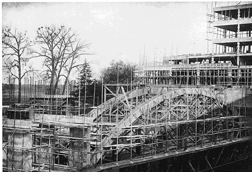
Figures 1.24 (a) and (b): Photographs taken during construction of La Cathédrale (Sauvestre, 1908) (top) and the passerelle connecting it to the rest of the factory complex (bottom), showing the scaffolding system for the Considère and Viennot reinforced concrete systems, c. 1906-8. (both © anonymous pictures – collection Ville de Noisiel)
