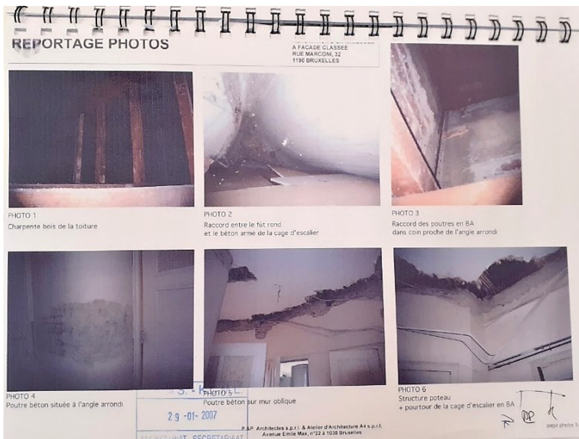
Figure 2.2: 2007 photographs of exposed (reinforced) concrete from a report on the structure of the HBM at 32 rue Marconi, Brussels (Govaerts, 1902), with no indication of the exact system used by the architect Govaerts. (FRT 2.51 CRM et Sites, Rue Marconi 32. Urban Brussels)
