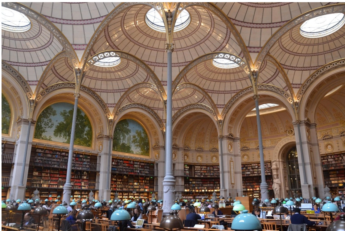
Figure 3.2: Modern day photograph of Henri Labrouste's reading room at the Bibliothèque Nationale, Paris (1868), with its iron pillars and delicate iron vaulting. (Adelphilos, CC BY-SA 4.0 via Wikimedia Commons)
