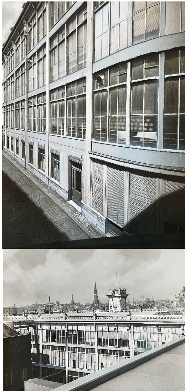
Figures 1.18 (a) and (b): Undated photographs of a facade with curved corner (above) and upper floors and roof terracing (below) of the early 'daylight factory' that was the Charles Six wool-combing mill, Tourcoing (architect unknown, 1897). (Peter Collins Fonds, John Bland Canadian Architecture Collection, McGill University Library)
