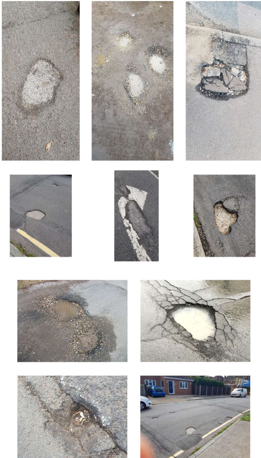
Figure 3.7: Supplemental dataset samples. These samples demonstrate the range of real-world conditions covered within the dataset. The demonstrated samples illustrate different challenging scenarios of pothole instances ranging from potholes located within road markings to rubble-filled potholes, water-filled potholes, rubble and water-filled potholes, and shallow potholes.
