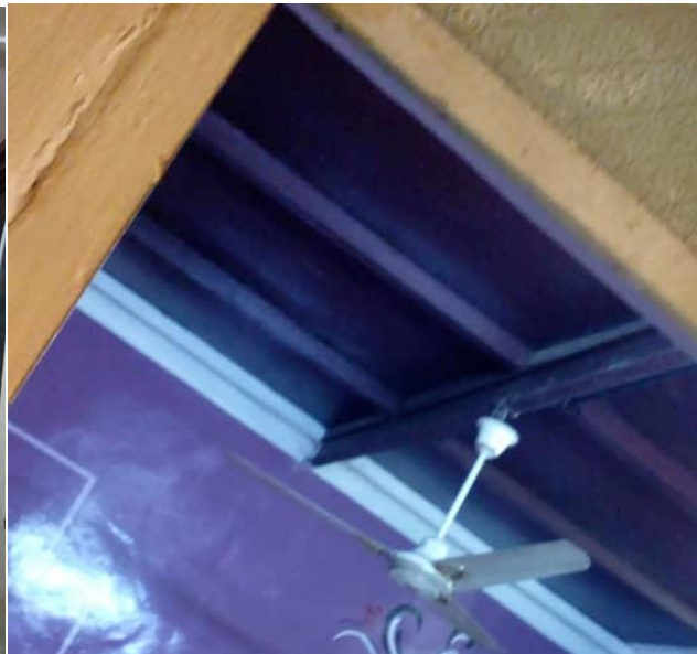
Figure 5.10 A photo of a wooden roof in T1
