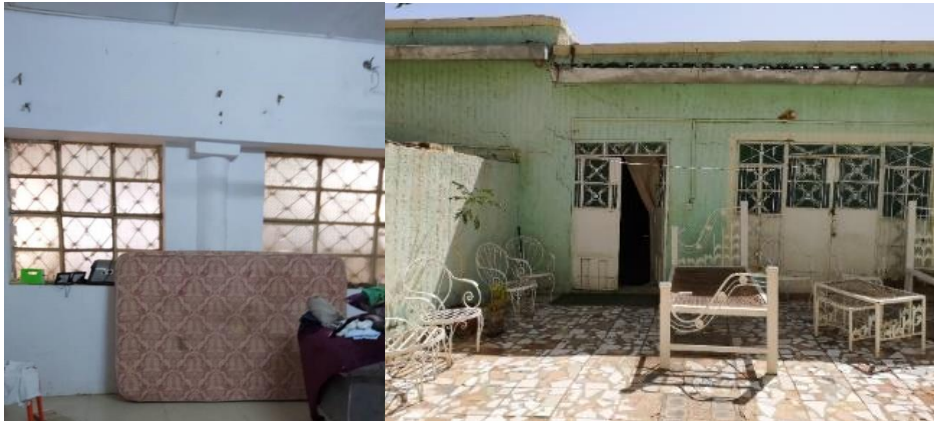
Figure 9.10 Windows and doors in converted verandas in the traditional houses T1 and T2
