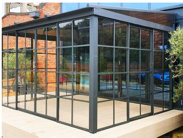
Figure 9.14 An example of a lattice metal bar secured patio
