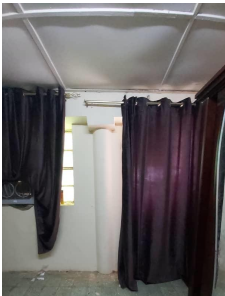
Figure 5.11 The original columns that held the veranda of the original house in T1
