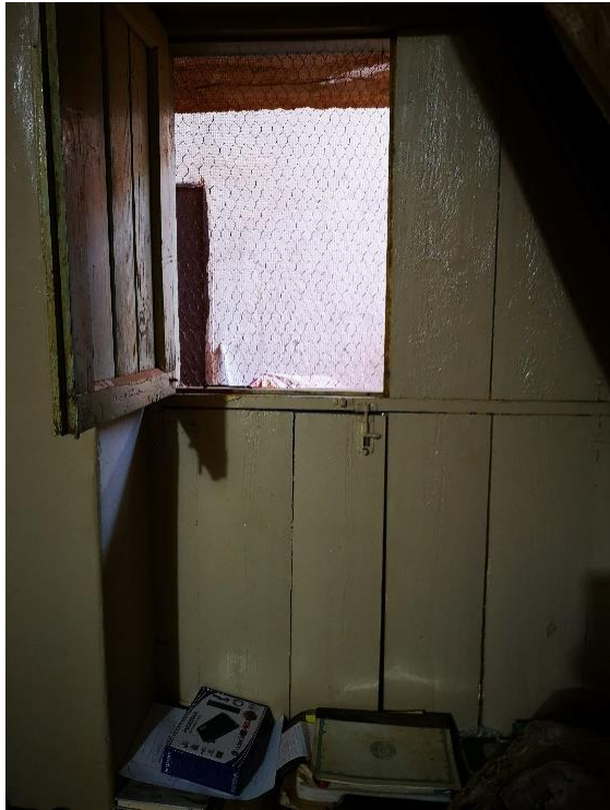
Figure 5.44 A traditional wood window with a mosquito mesh at T3
