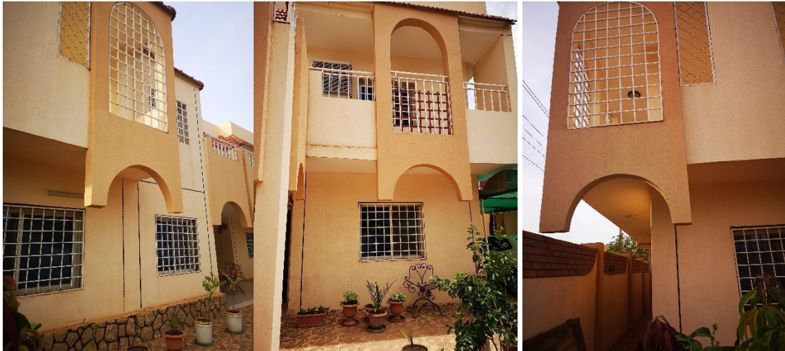
Figure 6.19 Balconies in M2 providing shade for the southern façade
