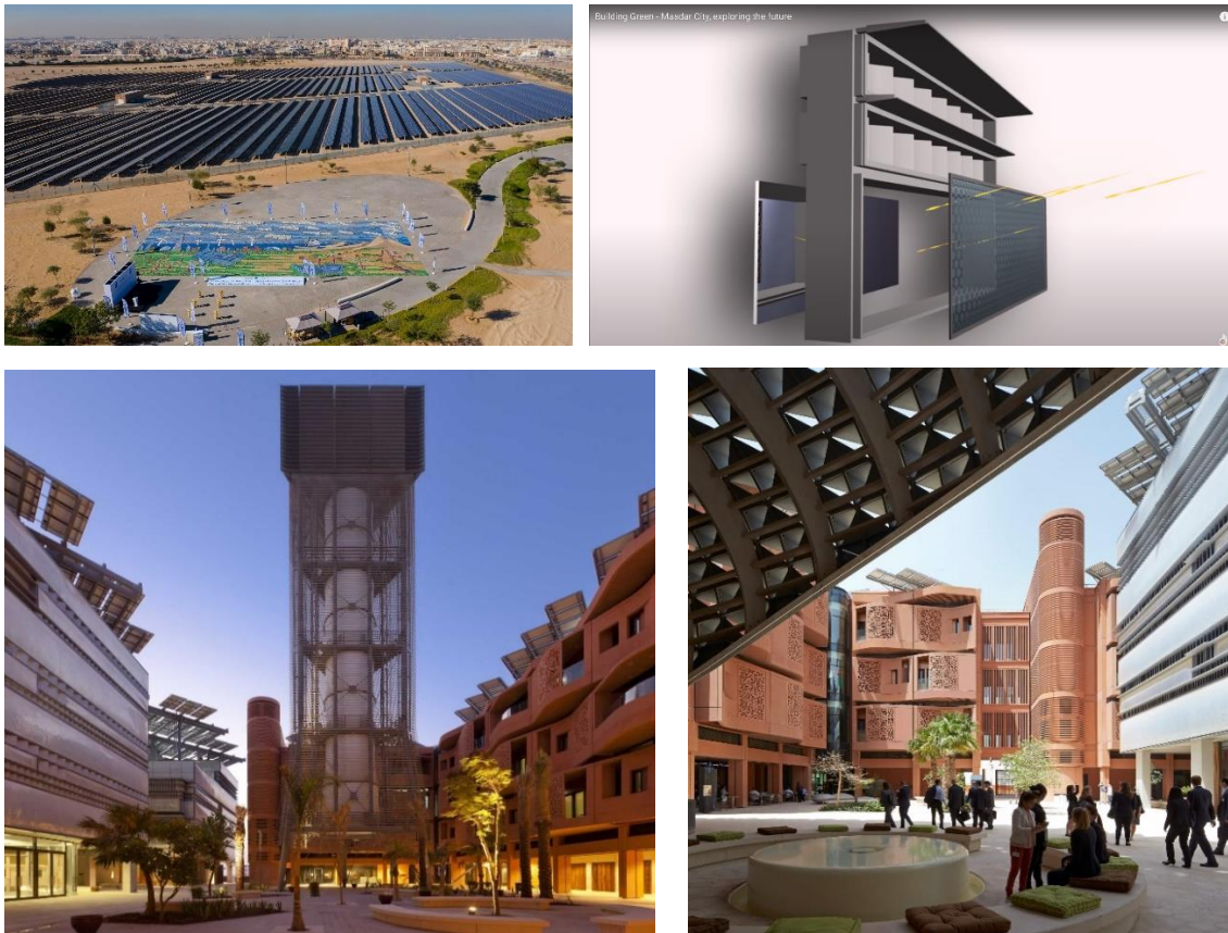
Figure 29 - 10 MW solar farm inside Masdar City (top left), ETFE panels used as insulation and shading (top right), wind tower (bottom left), courtyard and façade design (bottom right)
