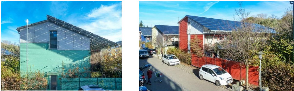
Figure 16- Side elevation of house showing shading from solar panels (left), view of internal road (right)
