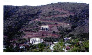
c) Road construction without erosion control, above Witches Brew, Tortola, 2002. Such practices accelerate sediment deposition in salt ponds
