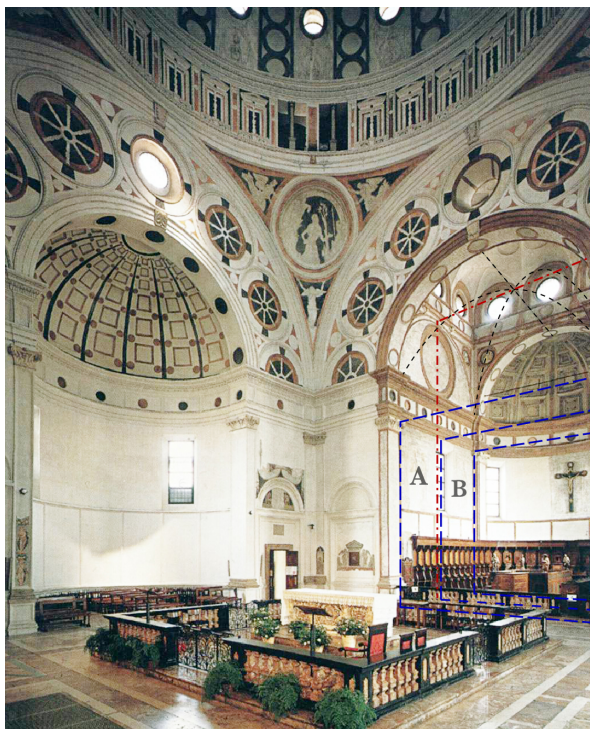
5.13—Santa Maria delle Grazie, Milan. View of the choir-sepulchral chapel with highlighted the different three-dimensional spatial sections (A, B) determined by the position of the choir's windows and final apse. Central axis of the choir's depth (905 cm) highlighted in red. Hypothetical crossing vault dotted in black.
