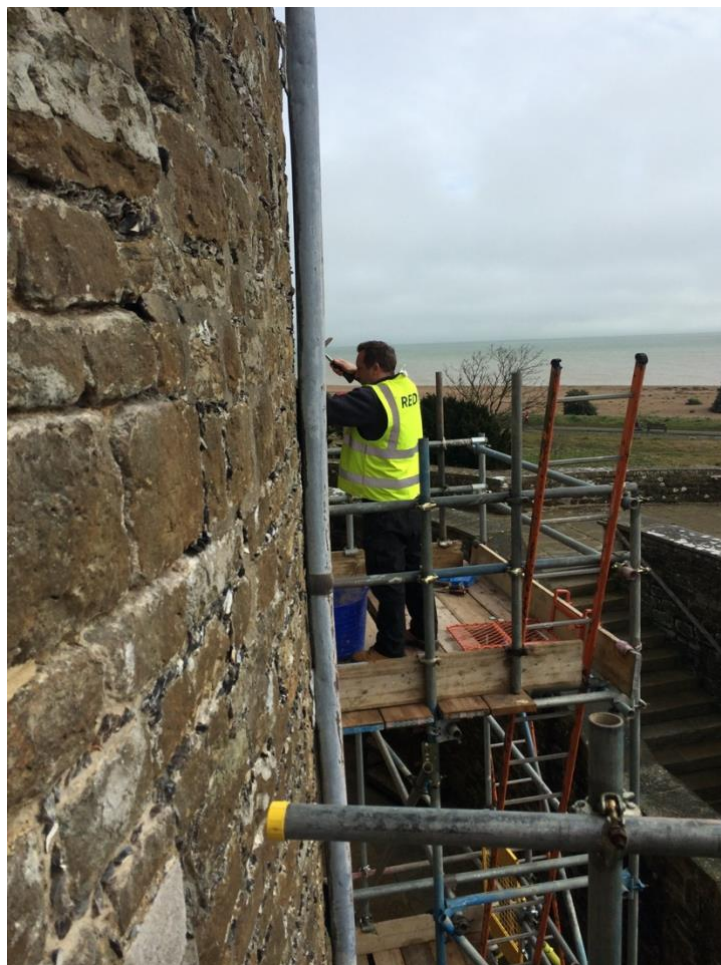
Figure 35. Conservation repair works to Walmer Castle, 2017 © Christopher Moore
