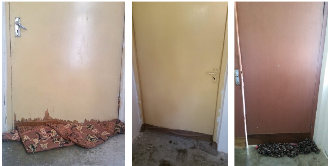
Figure 7.38 The way the household deals with air leaks through the bottom of the doors (author)
