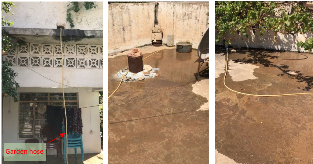
Figure 7.37 The garden hose taken to the rooftop to reduce heat gains through the roof and promote evaporative cooling around the house (author)
