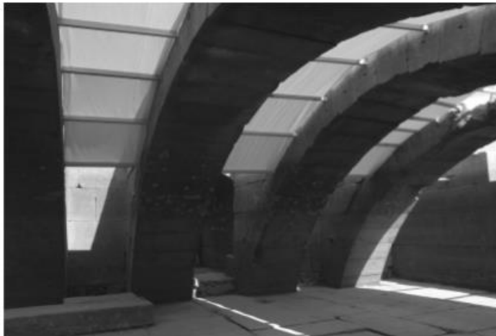
Plate 31 View of the restored battens and fabric covering in the adyton from the inside, southeast (Moretti et al. , 2011, 293).
