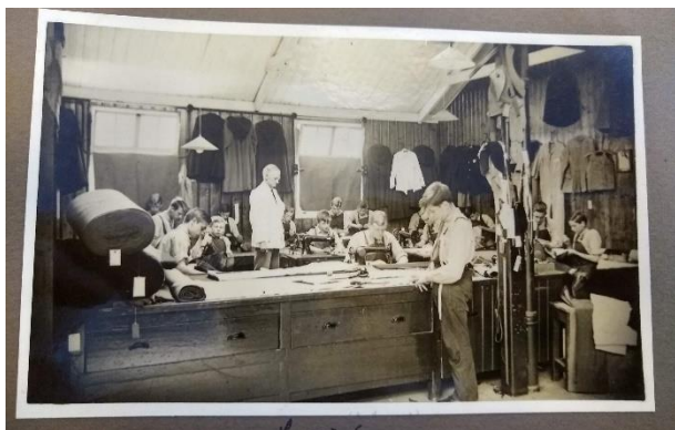
Figure 3: Boys tailoring in the workshops at Treloar College, Alton. c. 1930s
