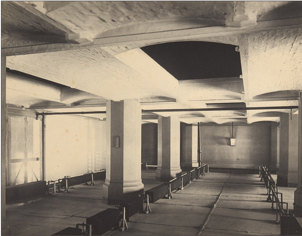
Figure 3: Interior of the air chamber, July 1897, showing canvas screens (left), three rows of heating batteries and apertures to the equalising chamber above.
