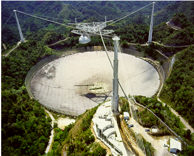
Figure 2.10: An image of Arecibo Observatory, a radio telescope located in Puerto Rico. The telescope is equipped with an S-band transmitter, which is centred at 2380 MHz - roughly 13 cm in wavelength. This facility is the second largest single aperture telescope with an aperture of 305 m. Image reprinted from NAIC Arecibo Observatory webpage.
