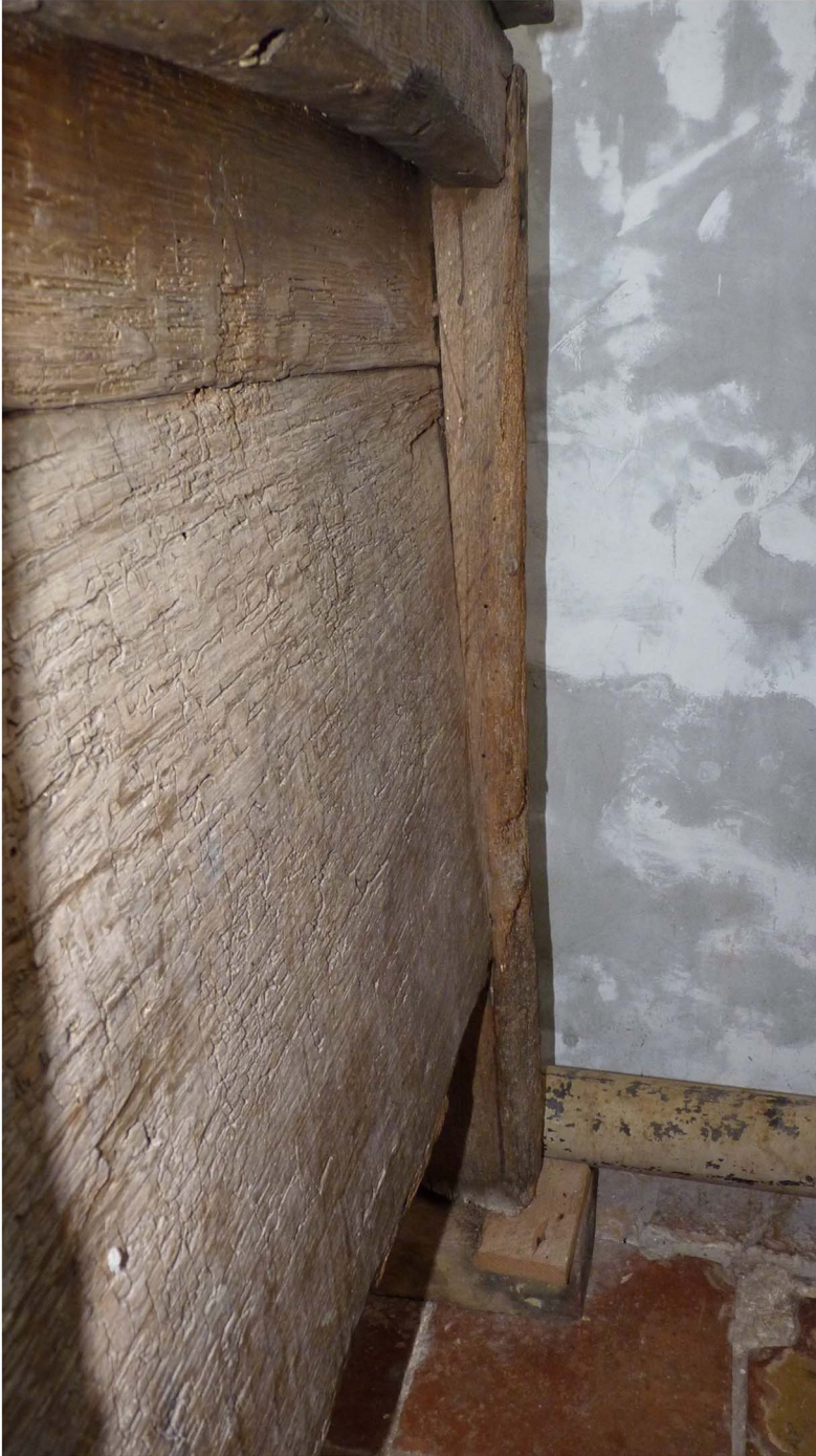
Fig 14. Inward-sloping sides allowing space for lid cleat within width of chest, Graveney. Photograph: author.
