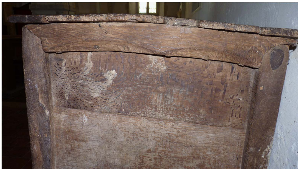
Fig 15. Protective plate over pin hinge and chamfered cleat, Wormshill. Photograph: author.
