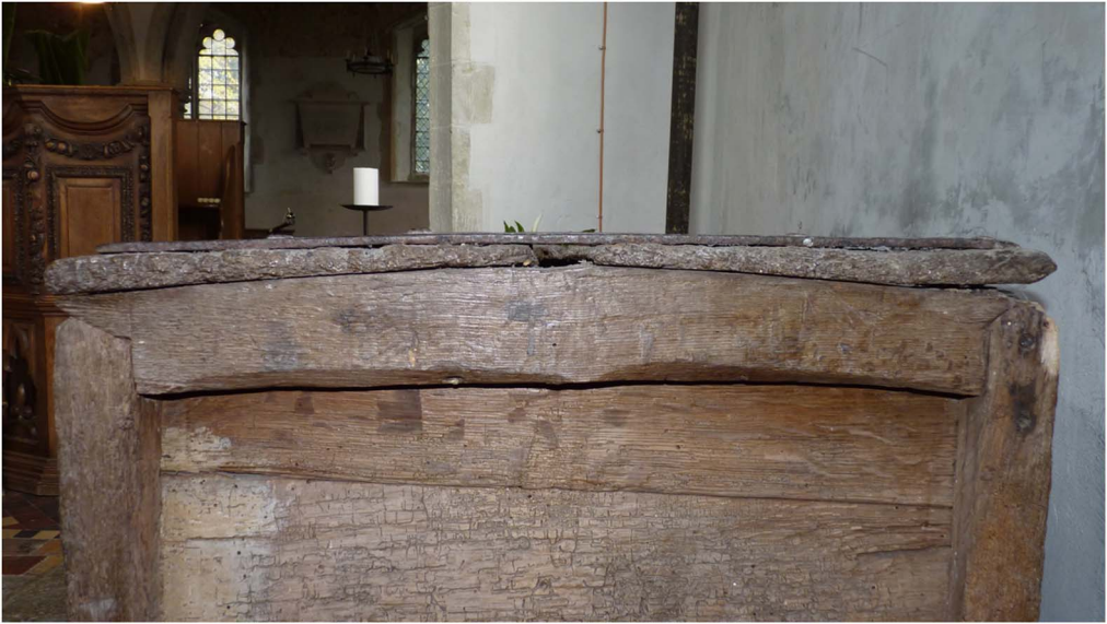
Fig 8. Side view of lid showing shaping of lid boards, cleat chamfers and shadow from protective plate over iron rod, Graveney. Photograph: author.
