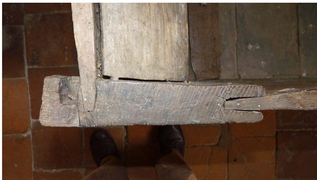
Fig 11. View showing tapered stile, notch for cleat and tapered tenons (and till box lid), Graveney. Photograph: author.
