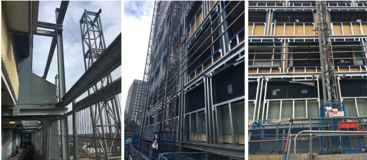
Figure 8.5. Skeleton installed to the courtyard façade (Photos by author, 2016).
