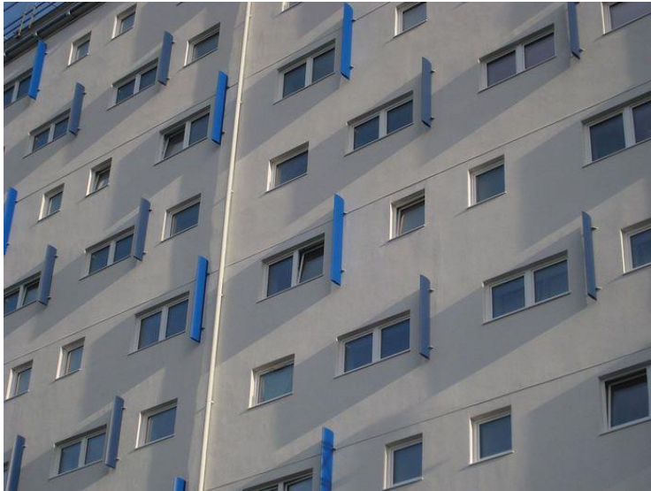
Figure 5.8. Vertical fins on the street façade (www.ribaj.com, 2018)
