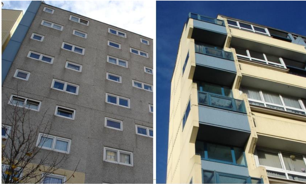
Figure 5.2. The photos on the left and the right show the street façade and the courtyard façade, respectively (ECD Architects, 2013).
