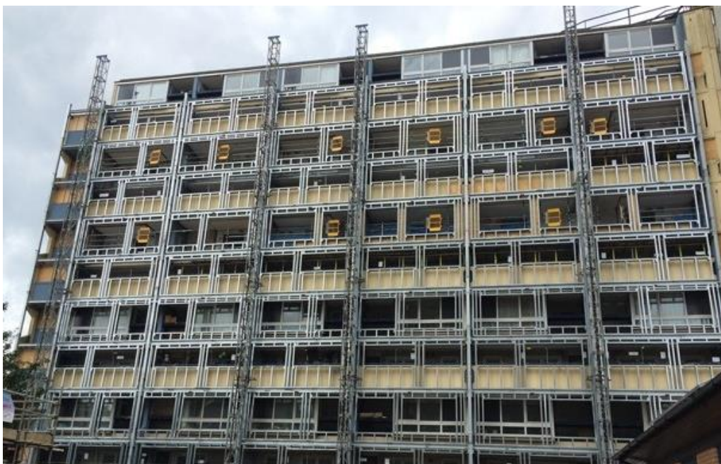
Figure 4.2. Steel framework and grillage on the rear façade of Wilmcote House (ECD Architects, 2016).
