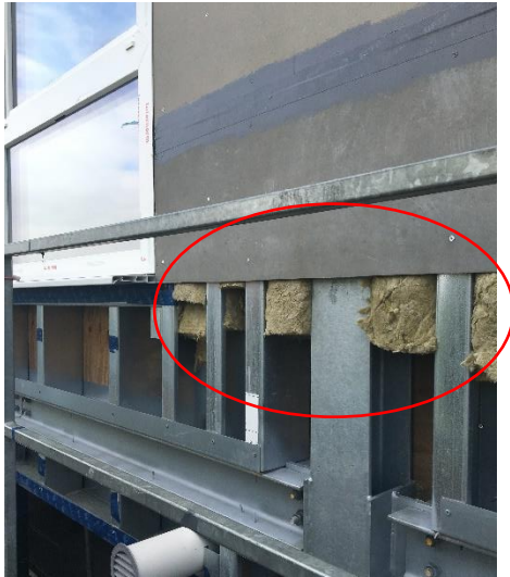
Figure 5.6. Insulation between the grillage channels. (Photo by author, 2016)
