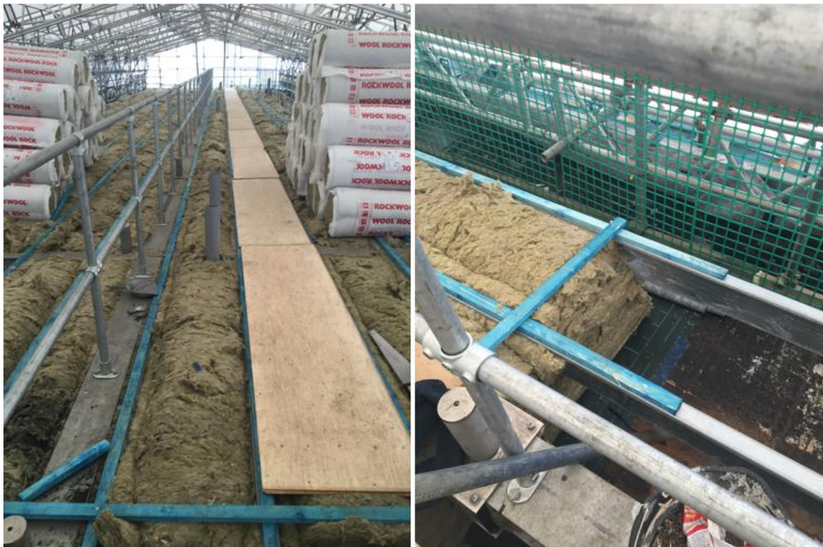
Figure 8.4. Insulation of roof and walls (Photos by author, 2016).
