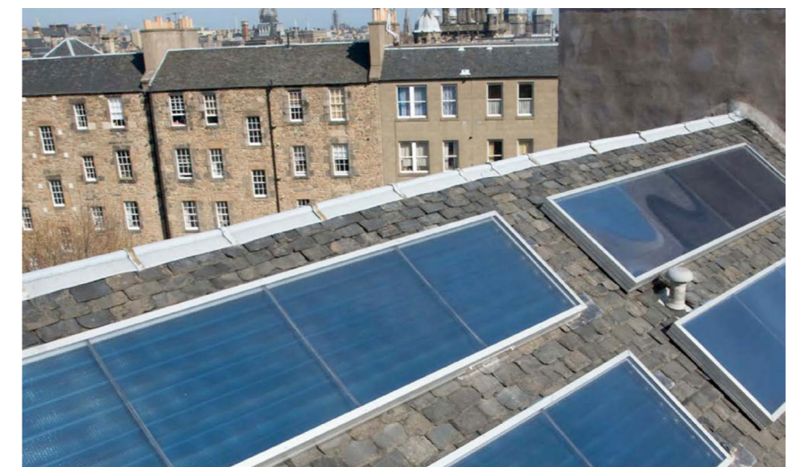
→ Solar thermal panels installed in a World Heritage site. (Historic Environment Scotland)
