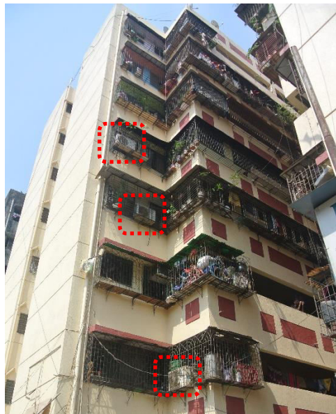
Figure 3: Multiple installed air conditioning units in Natwar Parekh Colony (photograph taken and annotated by Anika Haque, 2018)
