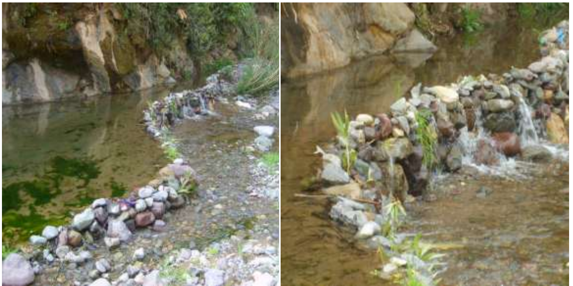
Plate 4.5 (a) and (b): Modifying river flow with dams and sluices to improve garden irrigation (El Maghzen, March 2008).
