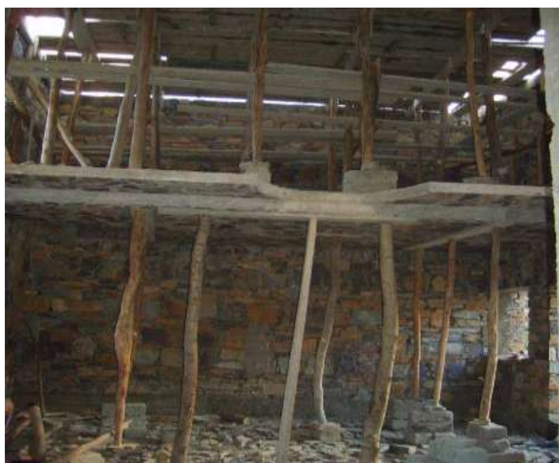
Plate 9.7: Building work started again after the INDH allocated a second sum of money to complete the building. This photograph also shows the internal floor to accommodate the alembic (El Maghzen, April 2008).
