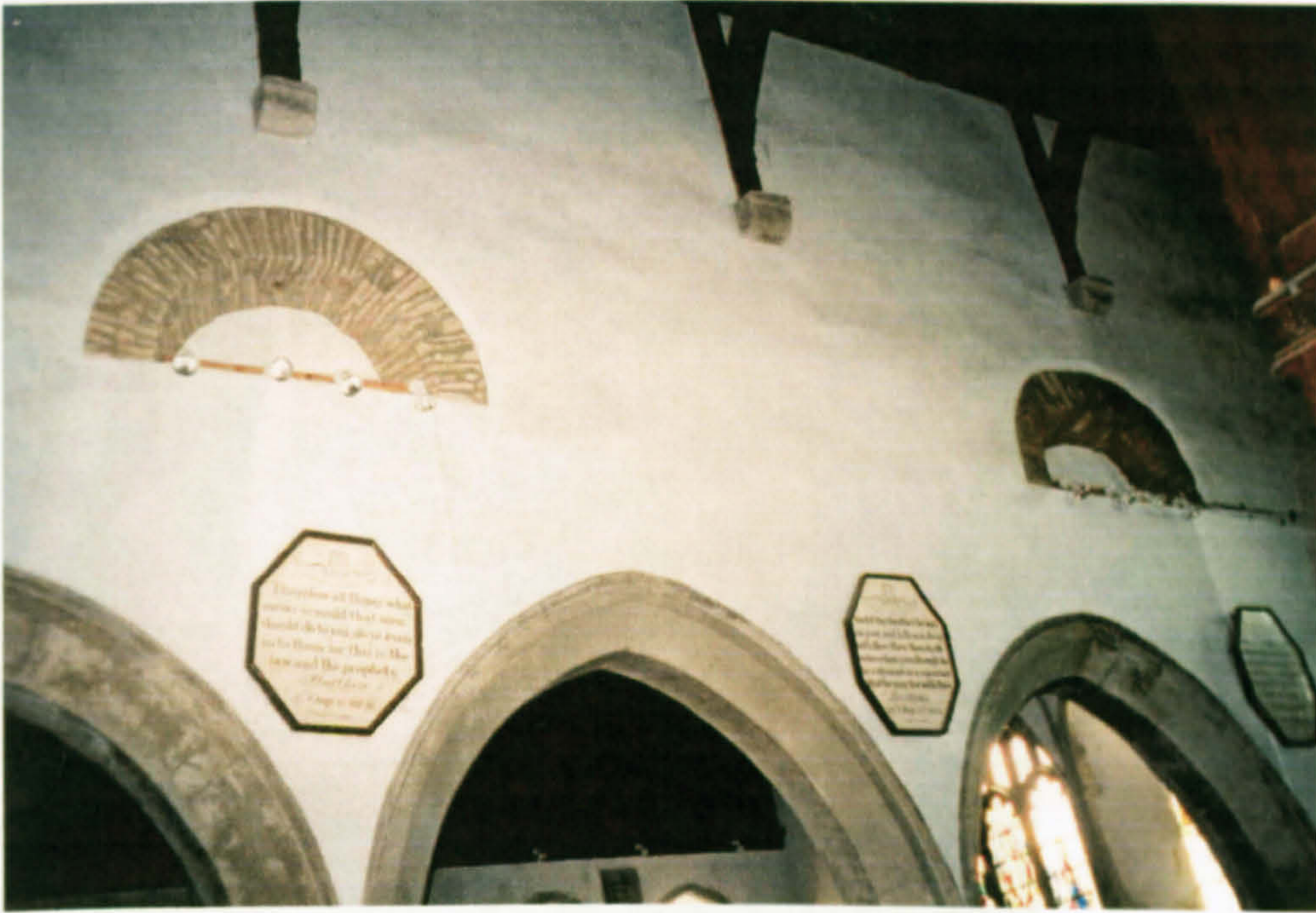
PHOTO 16: Evidence of earlier Norman windows in middle wall which may have divided the two monastic and parish churches of what is now the parish church of Minster.
