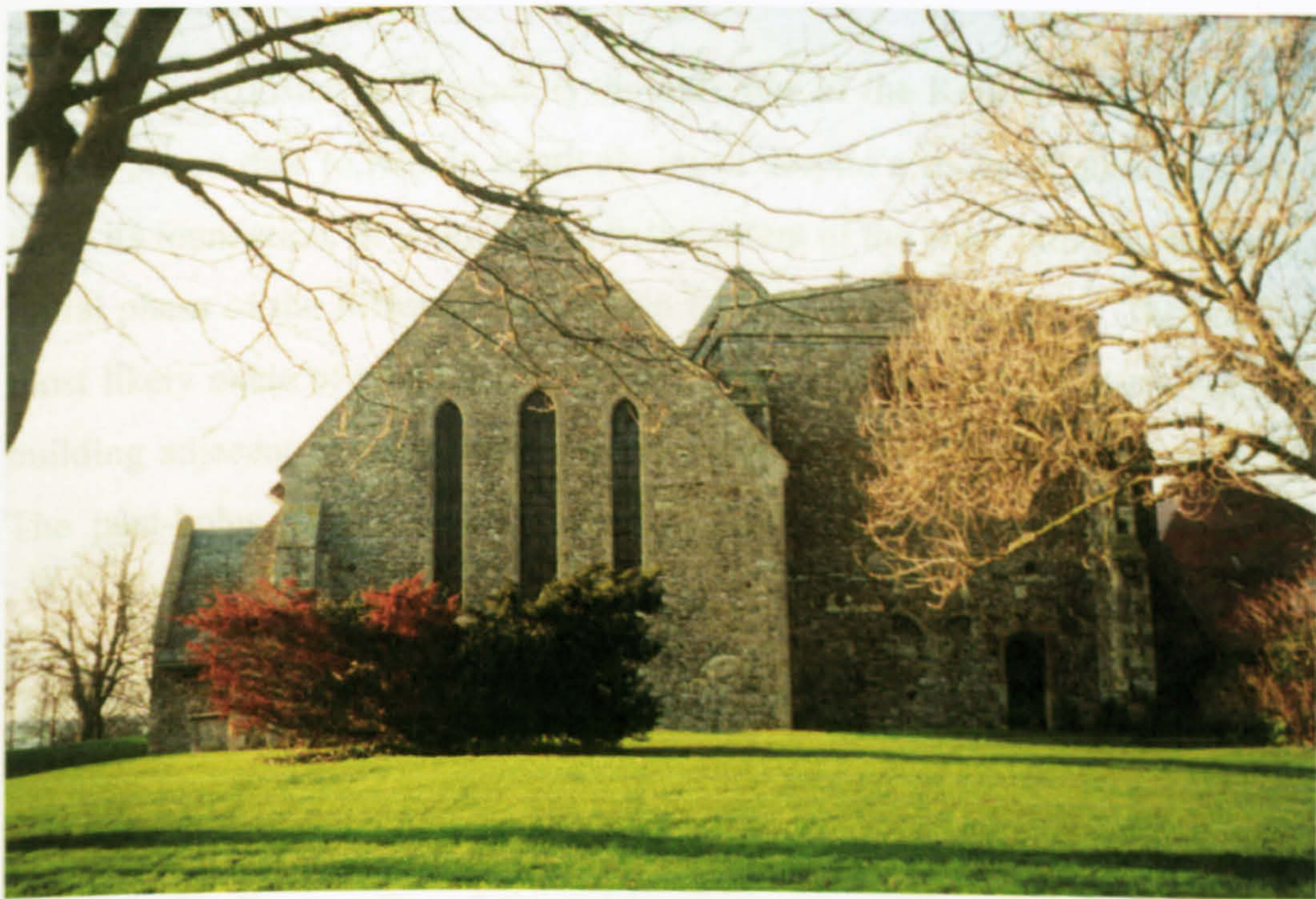
PHOTO 14: SS Mary and Sexburga Abbey and Parish Church, eastern approach. Evidence of Anglo-Saxon monastic church on the far right exterior wall with early arches still intact.
