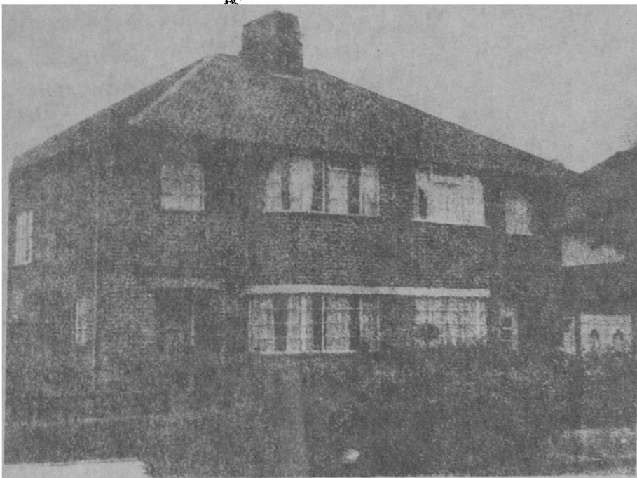
D Houses (Canons) Ltd Howberry Road, Edgware. 1935-7
