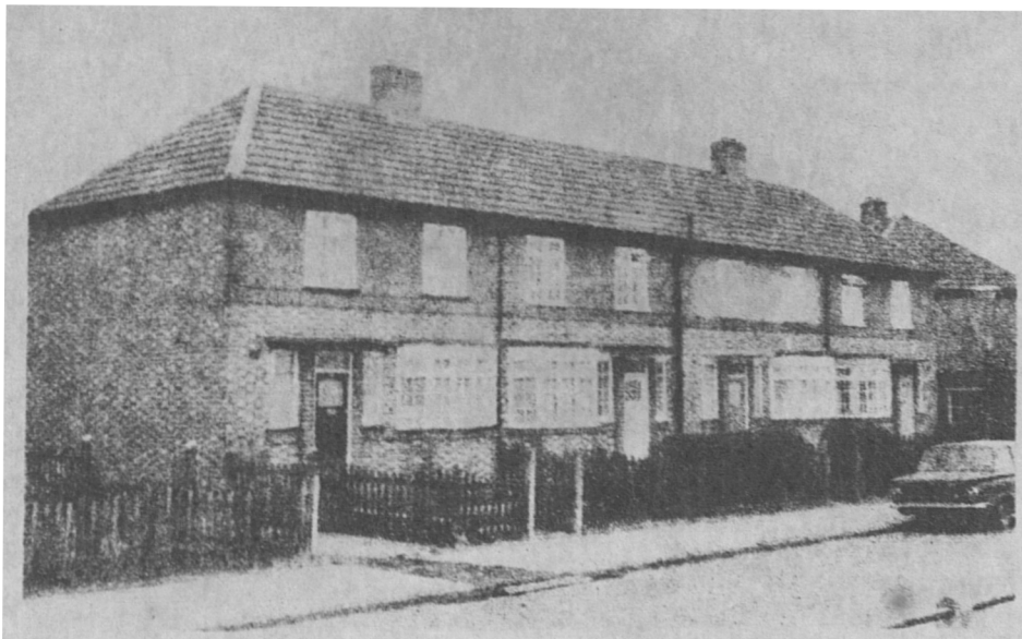
Queensbury Road, Alperton. 1934-6
