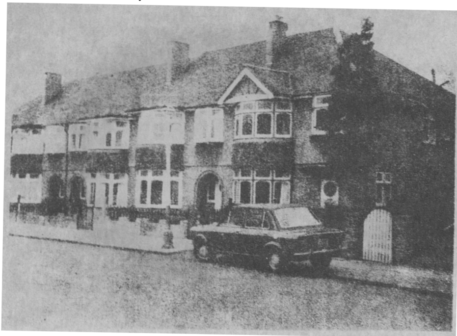
London & Provincial Building Co Ltd Brunswick Road, Ealing. 1931-3
