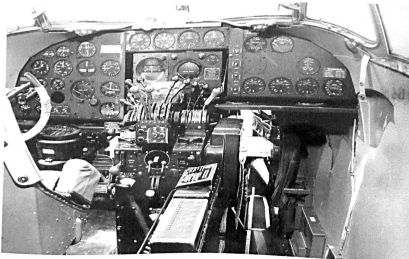
3. The wireless operator's view on the Hudson flight deck that had about 100 instruments and controls to be considered. Both the wireless operator and navigator could be expected to help the pilot in landing at such as Gibraltar in respect of flaps and undercarriage.
