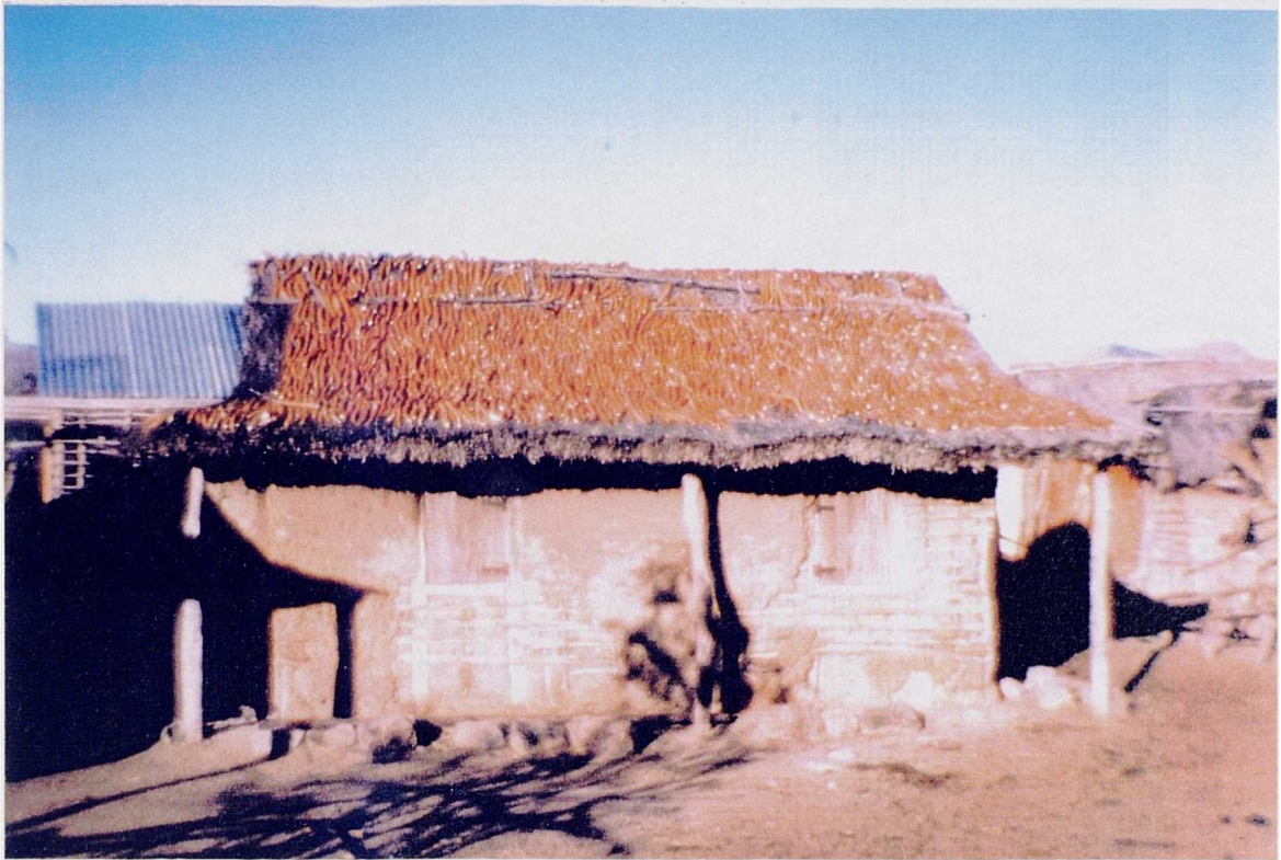
Figure A12.14 House in Esomony. The frame is made from wooden posts and the walls are plastered with mud. Manioc ( Manihot esculenta ) tubers are drying on the roof.
