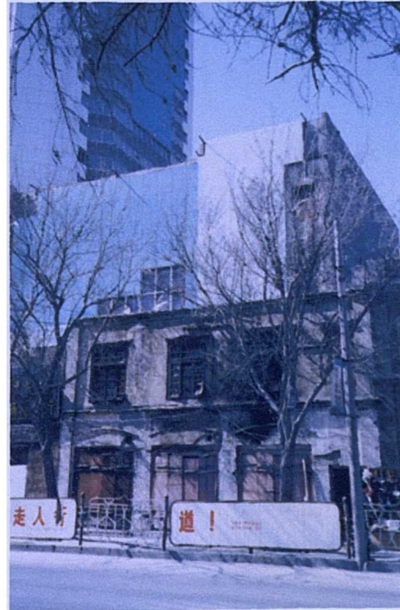
Photo 17 An old building on Jiefang nanlu . Behind, a new building under construction.
