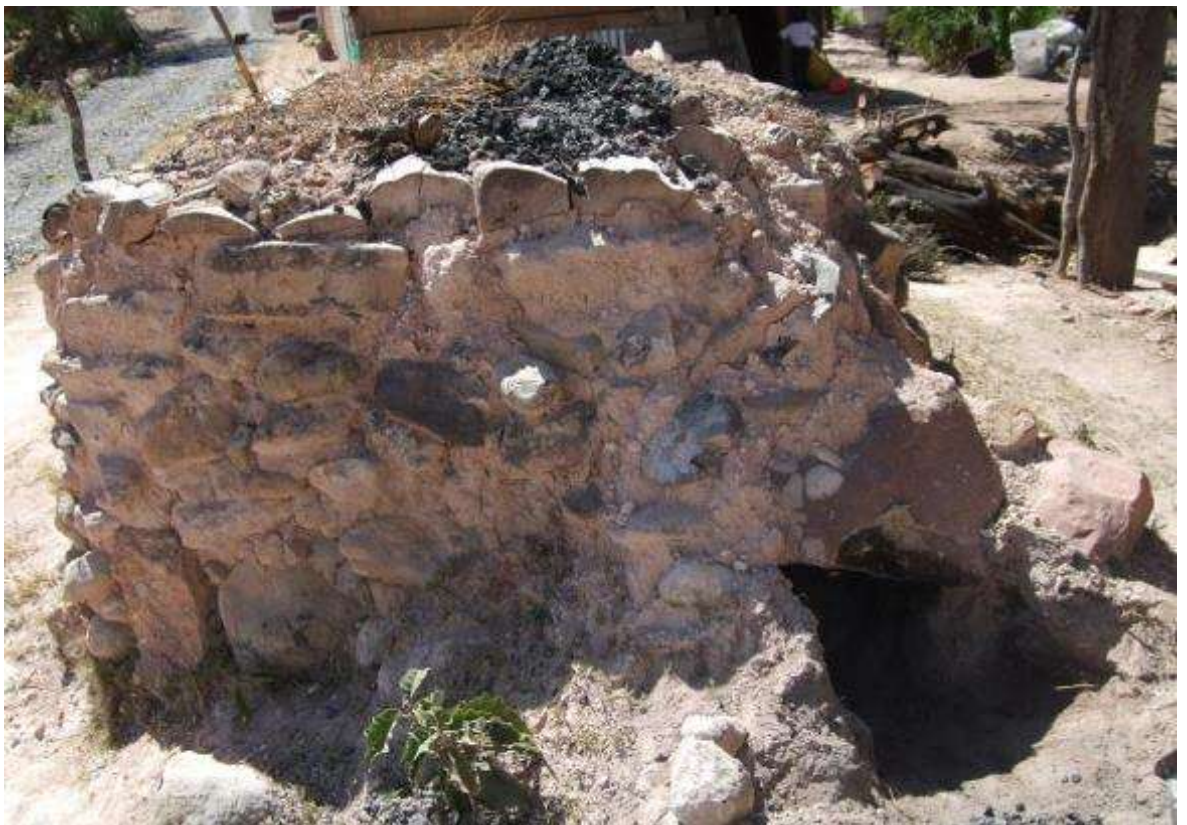
Figure 6.5: This is the back of the temazcal with the ndaka ñi'i or hornillo opened up on the right.
