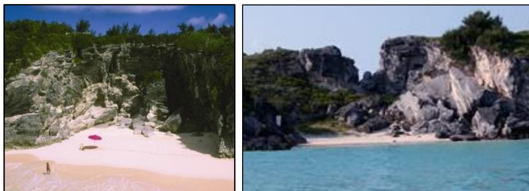
FIGURE 1.7. Rock fall on Charles Island (before and after) following hurricane Nicole in 2016. (Photo Credit: Dept. Conservation Services. 2000; Turner, H. 2016).
