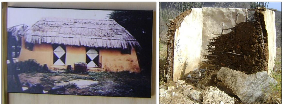
Figure 6.6: Display panel at the Kas di Pal'i Maishi showing traditional kunuku house (left) (image courtesy of the Kas di Pal'i Maishi ); and an example of wattle and daub construction at Plantage Kenepa (right) (Source: Author).
